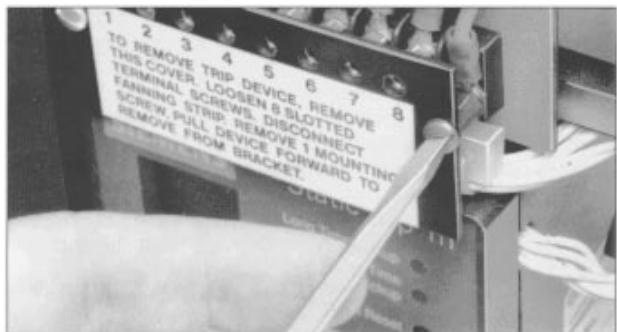
5.) Replace the terminal block cover.
