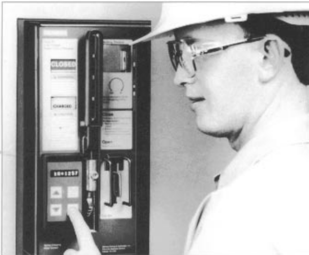
BDU Mounted on Type RL Circuit Breaker
