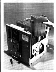
DS Breakers are designed for easy contact inspection and maintenance.
