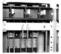
Welded aluminum busses and a coordinated glass polyester insulation system assure continued reliable operation throughout the life of the installation.
