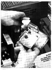
The stationary contact assembly is held by two readily accessible bolts at the rear of the breaker.
