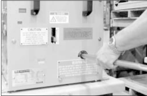
Figure 3. Manual Trip & Close
