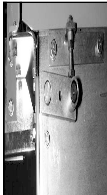
Figure 39. Positive Interlock
