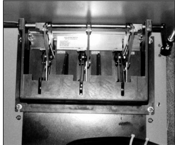
Fig. 10 Isolation Switch
