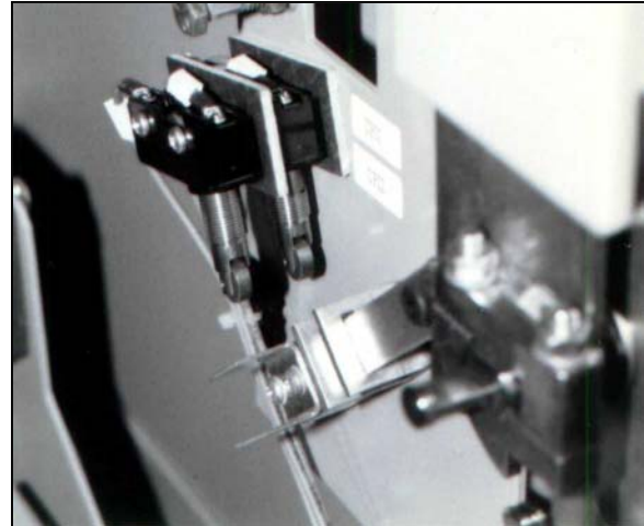
Fig. 9 Control Power Interlock
