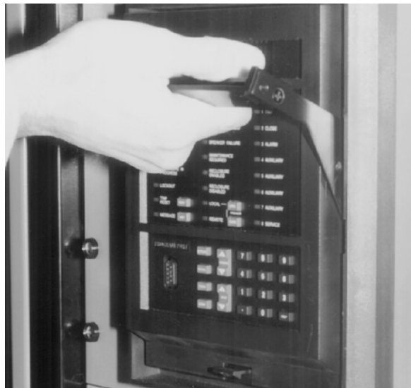
Figure 3-6: ROTATING HANDLE TO STOP POSITION
