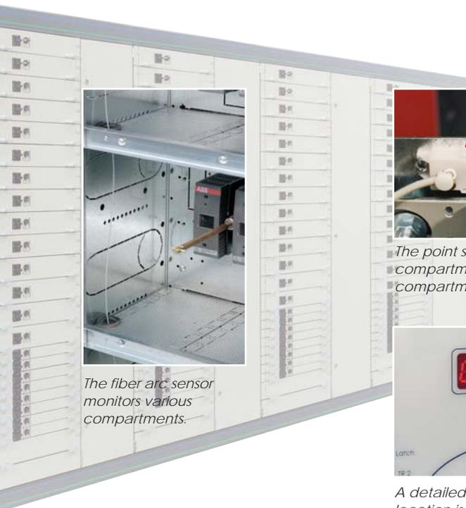
The fiber arc sensor monitors various compartments.
